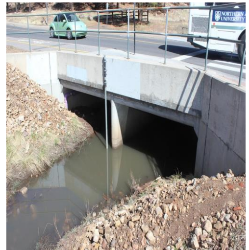
Figure 1.2.2b Culvert under South Knoles Drive
